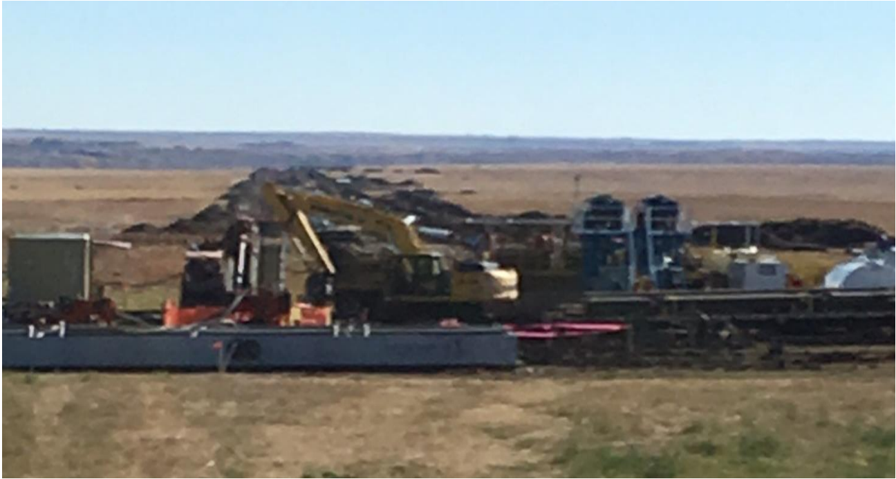
Canal Directional Drilling
