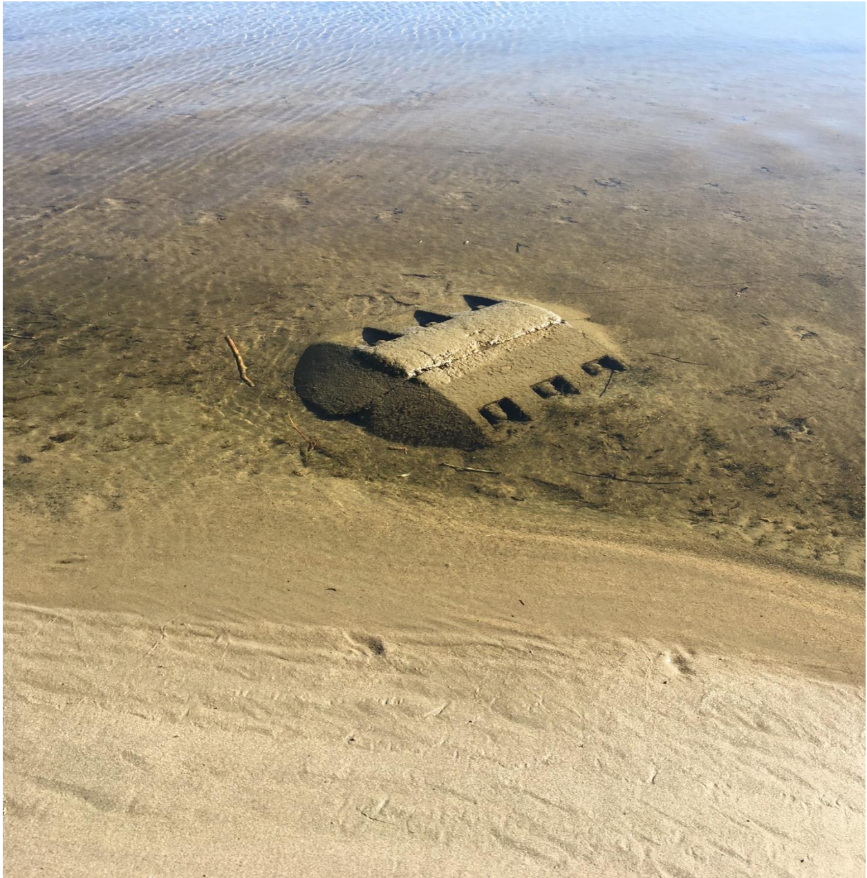
Appears to be a weight for an existing pipeline at the river
