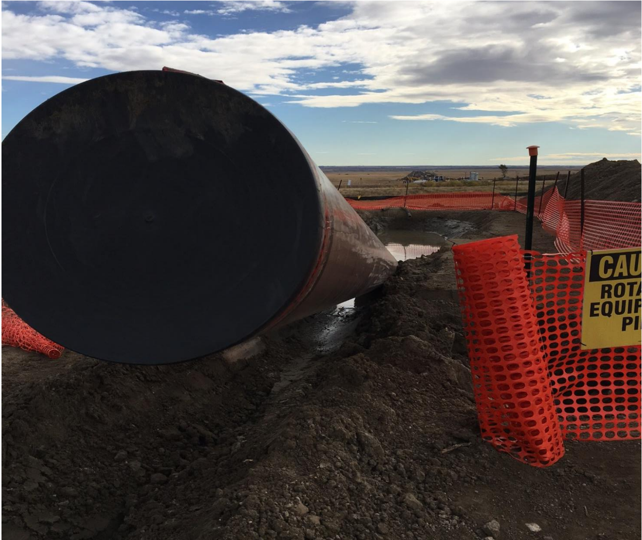
Pipe that has been pulled through at the canal
